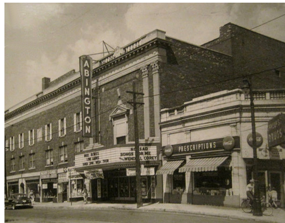
Figure 9: The building on Twelfth Street in Detroit that housed Littman's People's Theater from 1937 to 1944 operated as a movie theater under the name "Abington Theater" from 1945 to 1953. ( https://cinematreasures.org/theaters/2798/photos/32971 .)
